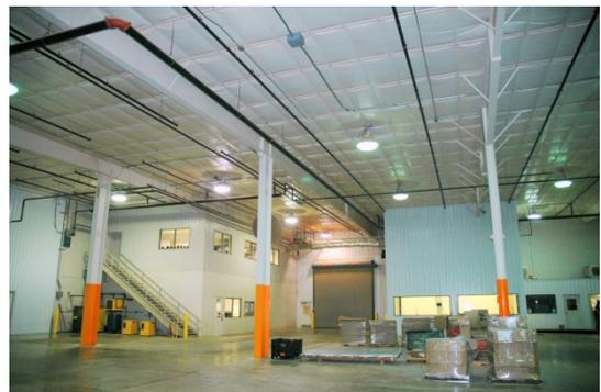
This warehouse uses a two-layer Filled Cavity (FC) system consisting of a first layer of fiberglass laminated to the vapor barrier that is installed from the top between the purlins supported by banding attached to the bottom flange of the purlin. The second layer is unfaced and installed over and perpendicular to the purlins with the thermal block above the purlin.
