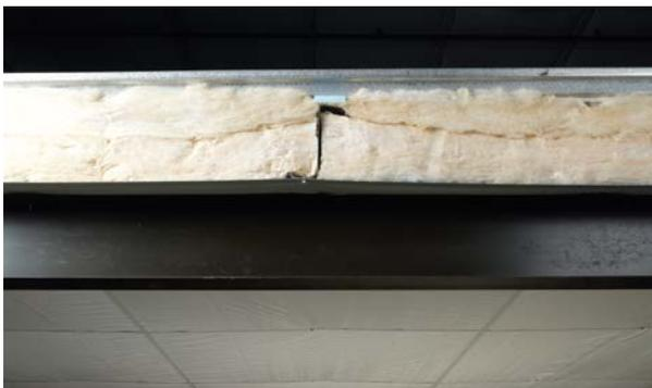
A cross-section of the Skyliner™ Liner System (LS) consisting of a single vapor barrier covering the entire bay, supported by banding at the bottom flange of the purlin. The first layer of fiberglass is installed in between the purlins supported by the vapor barrier. The second layer as with the LTB system is installed over and perpendicular to the purlins with the thermal block above the purlin.
